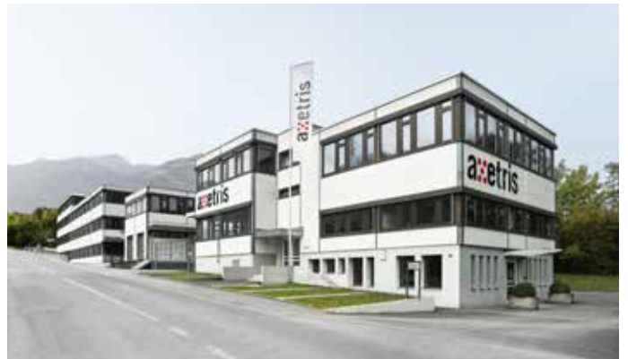
Leister Technologies AG, factory, Kaegiswil, Switzerland
