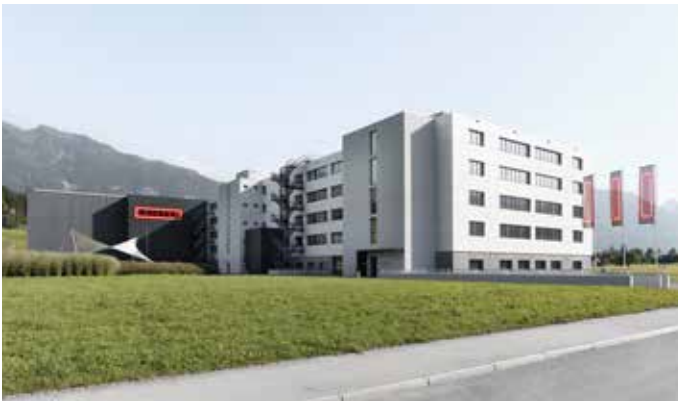
Leister Technologies AG, factory, Sarnen, Switzerland
