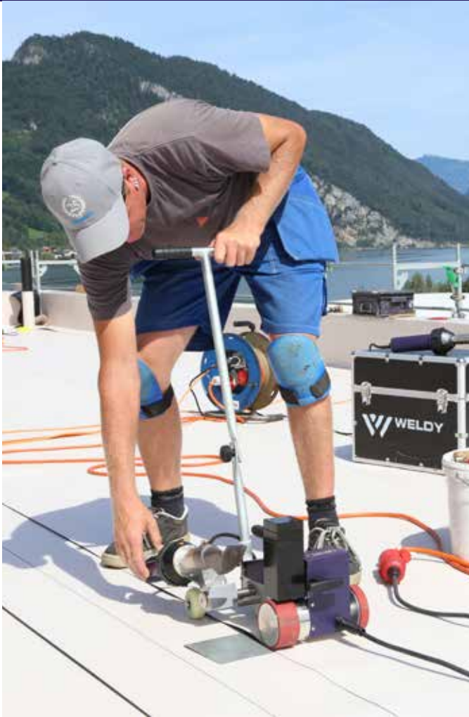
123.287 Overlap welding nozzle, 40 mm
